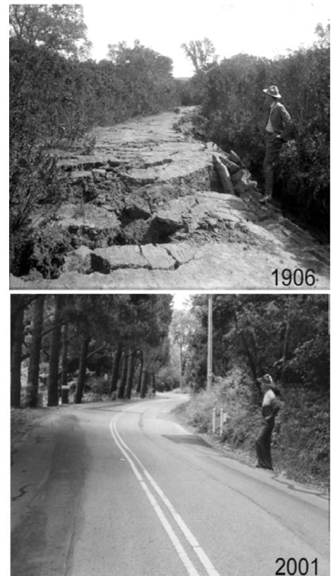
*The 1906 photo, shown here for comparison with a modern photo at the same location, illustrates the 6-foot displacement of Alpine Road and sheds some light on what to expect in the next such earthquake on the fault.*
