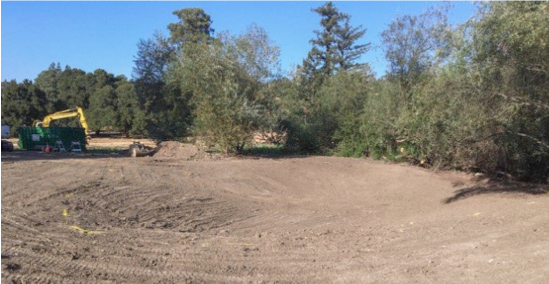
12. Final Pond Grading
