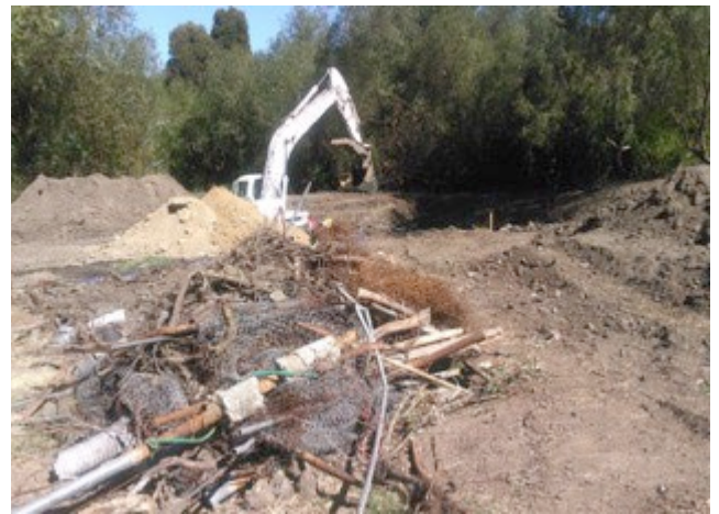
9. Clearing the old fence and other debris.
