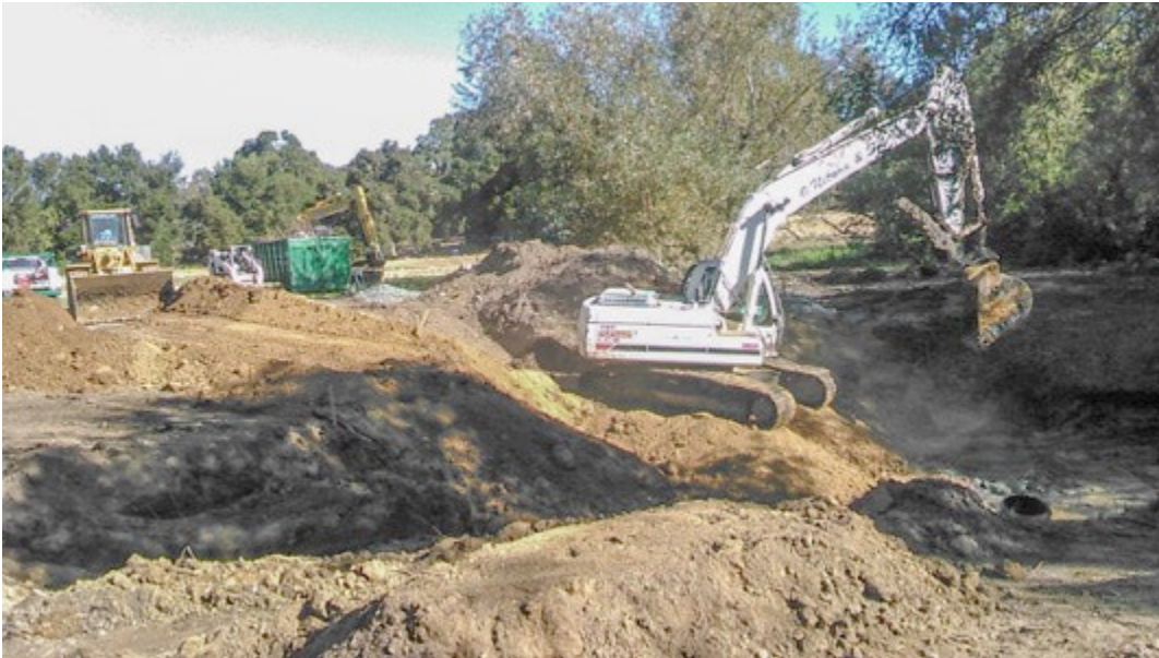
10. Excavation equipment –two graders and two shovels.
