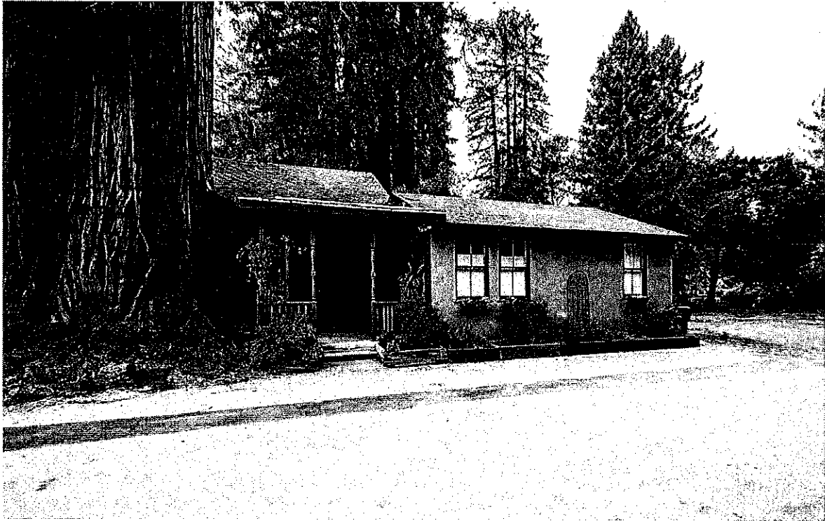
Northern portion of east façade, view looking west (Architectural Resources Group, March 2016)
