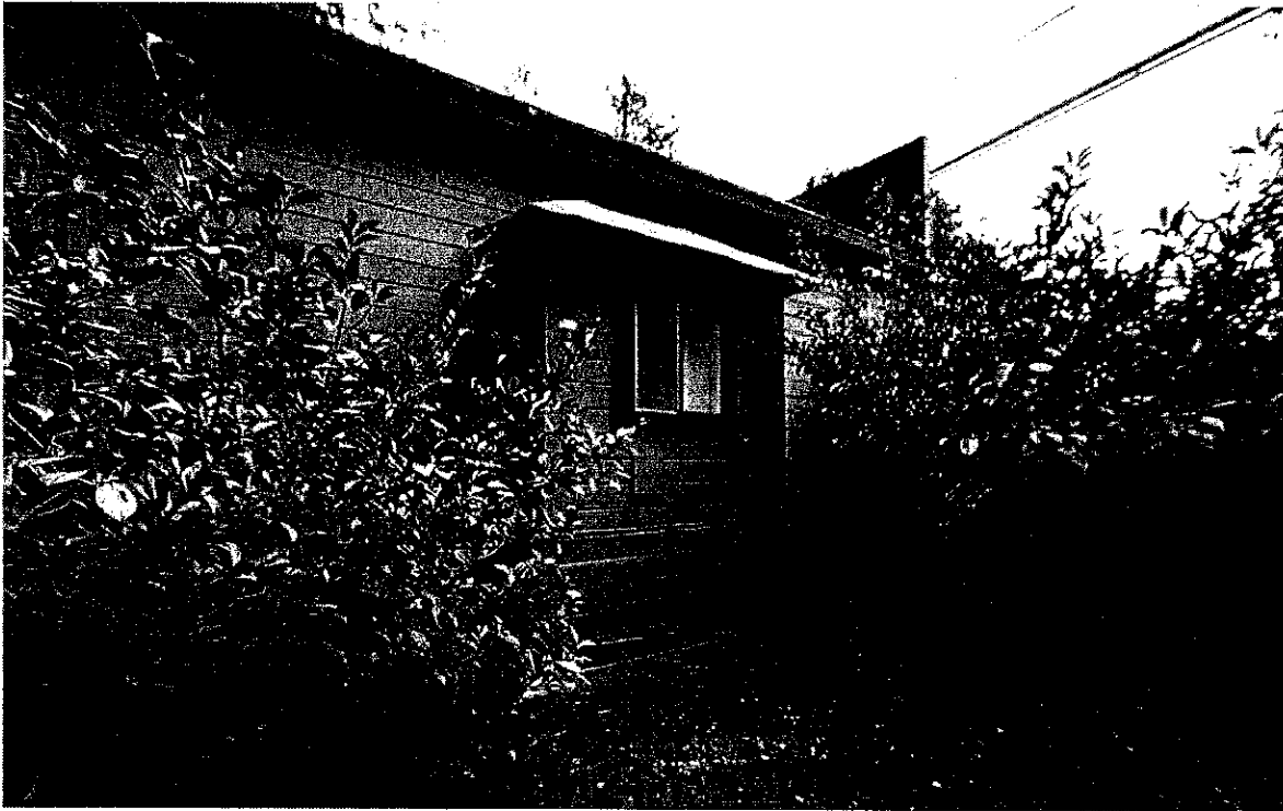
Southern portion of west façade (Architectural Resources Group, March 2016)
