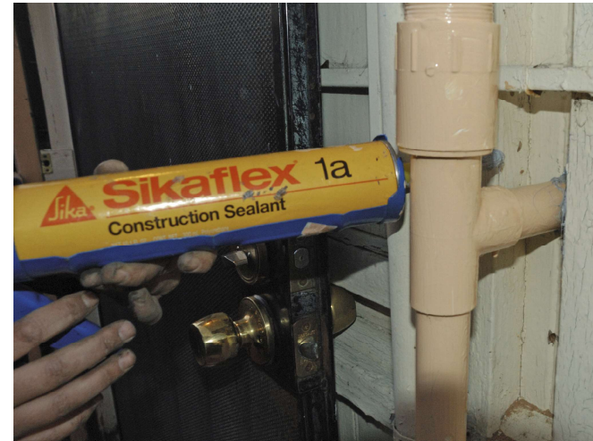
Exposed PVC pipe is painted to protect it from UV degradation. The hole is sealed with an adhesive sealant to prevent moisture from entering.
