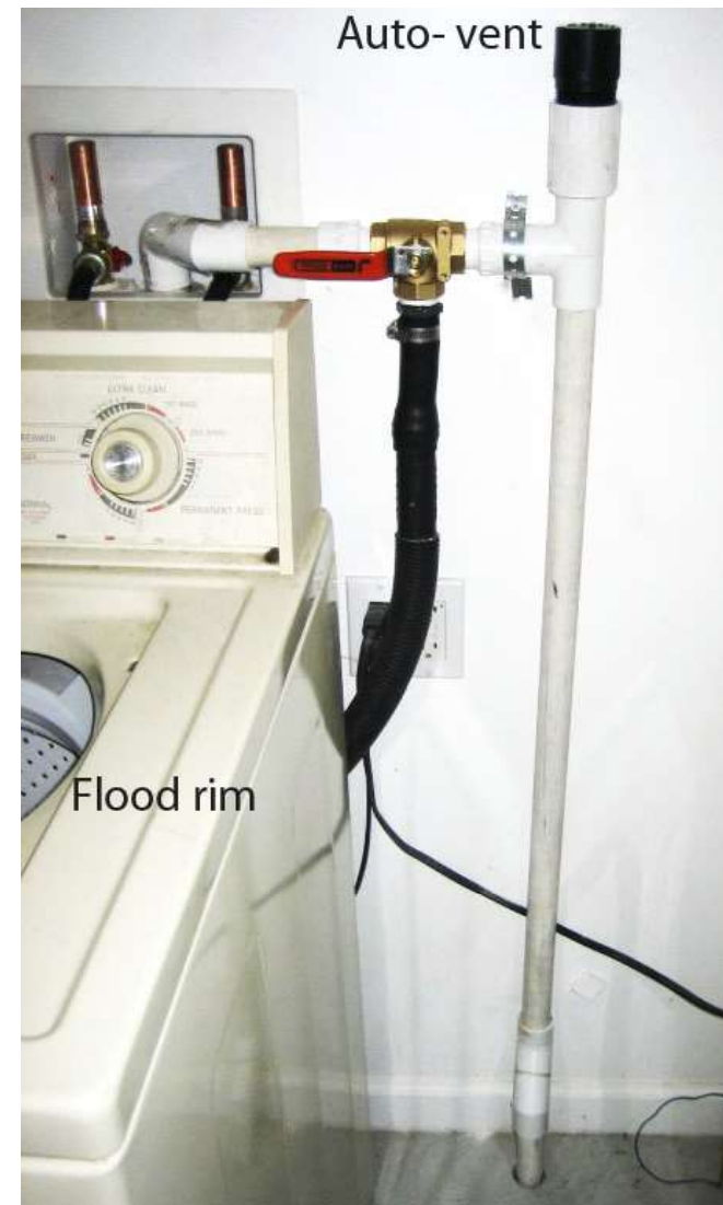
The 3-way valve is slightly above the sewer connection (behind the machine), while the auto vent is about a foot higher than the flood rim of the machine. (Floor installation with auto vent inside house) Photo: Laura Allen.
