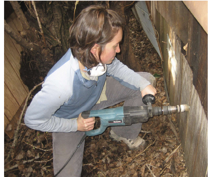
Drilling a 1½-inch hole for pipe. Note: A pilot hole was drilled first. Photo: Laura Allen.
