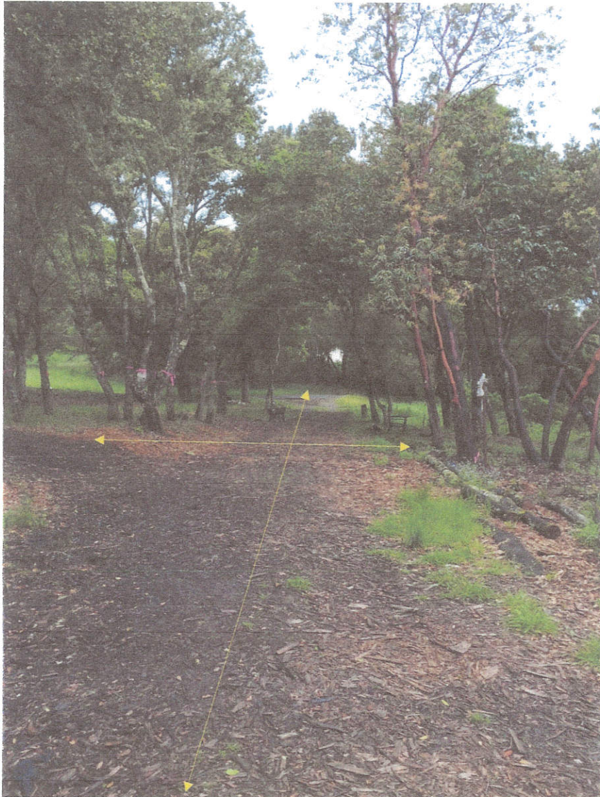
Tree inventory within easement along proposed driveway path, towards Wayside Road. Yellow arrows indicate length and proposed width of 30' for construction.
