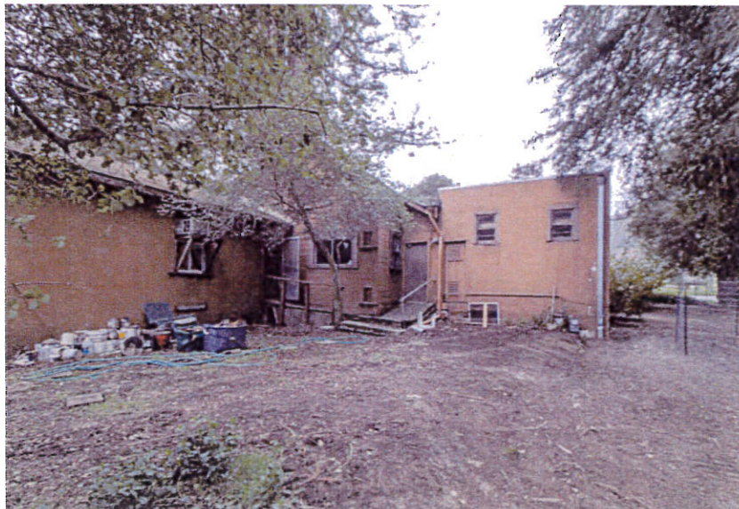
West and north façades (Architectural Resources Group, March 2016)
