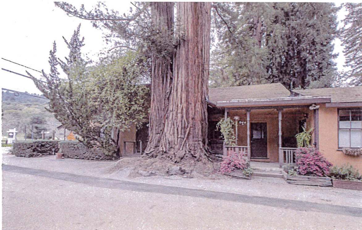
Southern portion of east façade, view looking west (Architectural Resources Group, March 2016)
