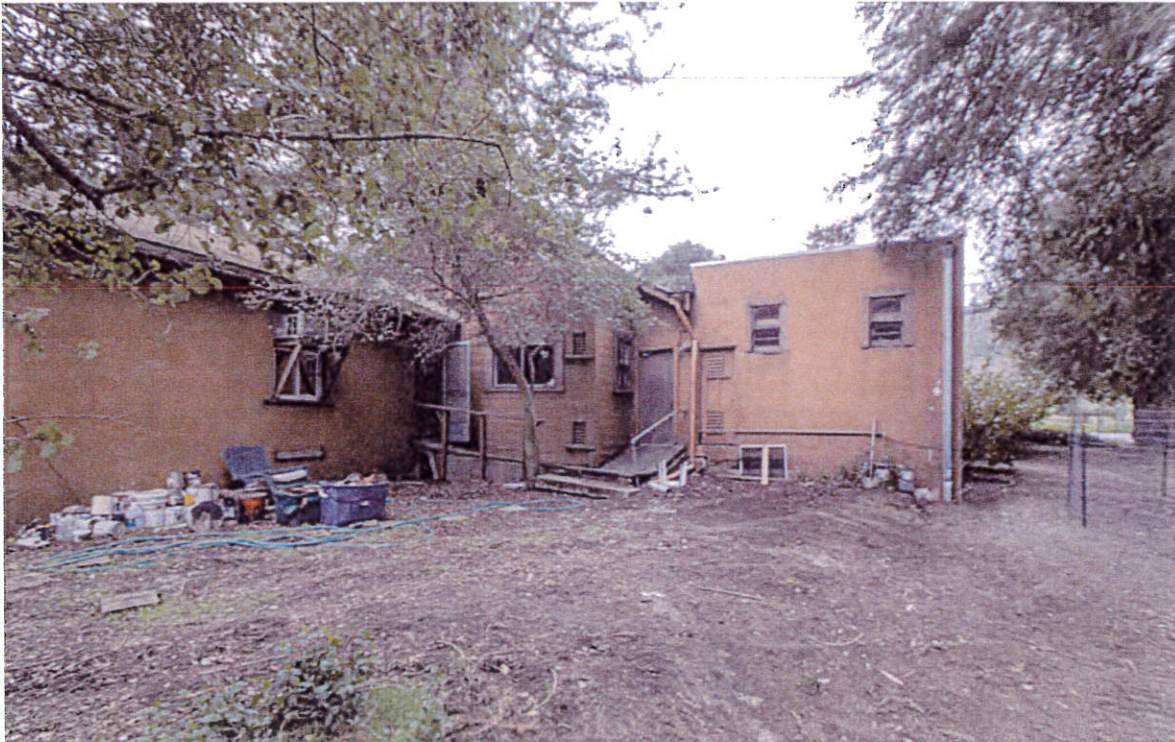
North and west façades, view looking southeast (Architectural Resources Group, March 2016)
