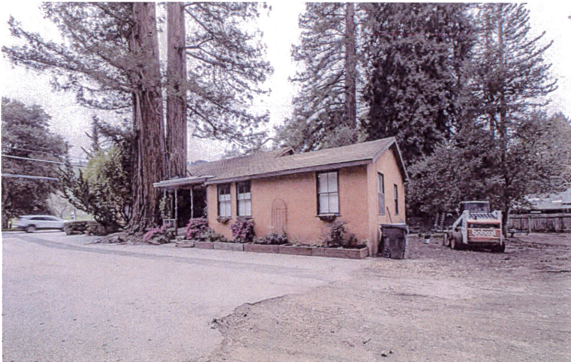
East and north façades, view looking southwest (Architectural Resources Group, March 2016)
