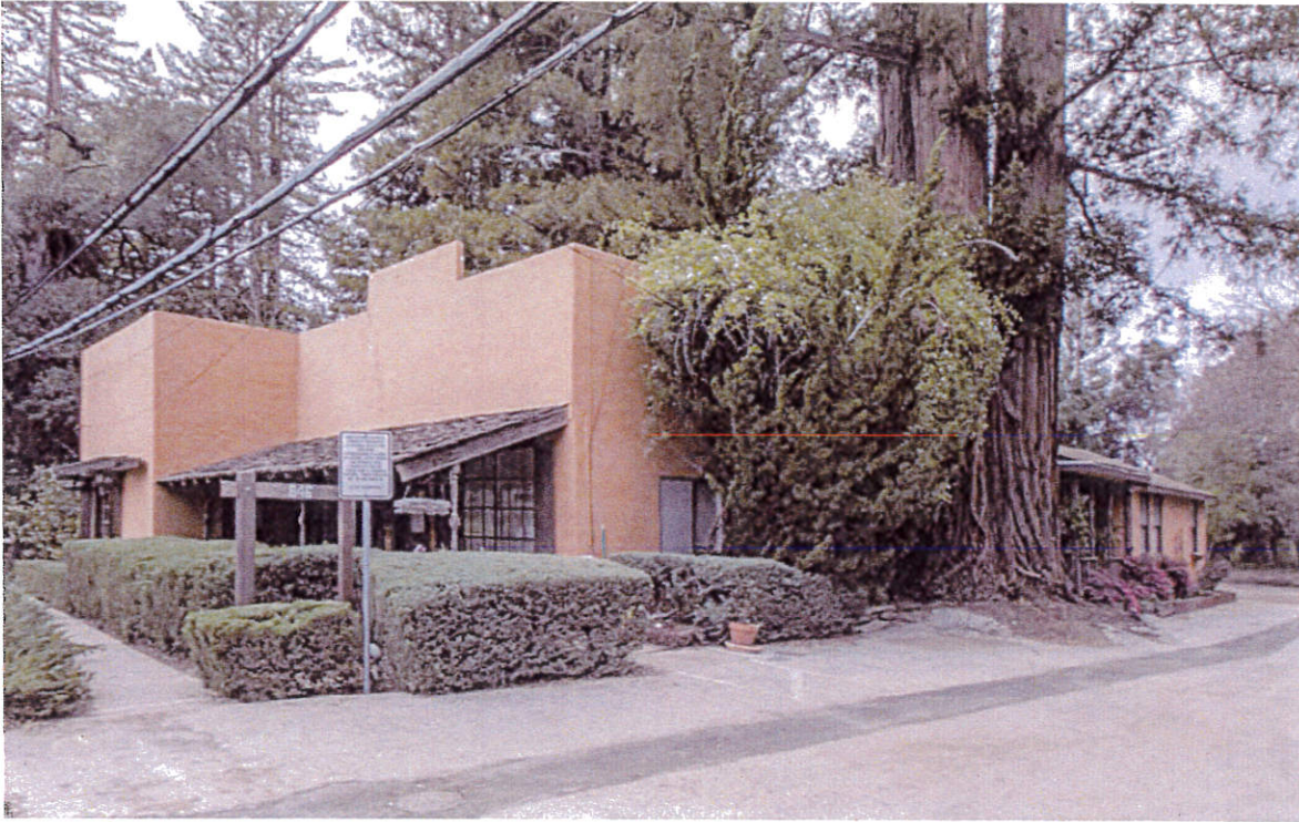
South (primary) and east façades, view looking northwest (Architectural Resources Group, March 2016)
