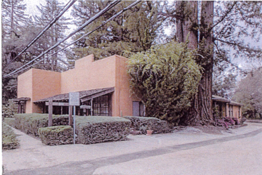
Primary (south) and east façades (Architectural Resources Group, March 2016)
