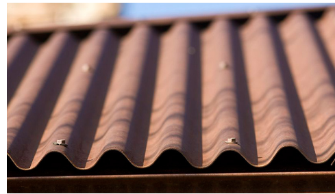
ROOF MATERIAL: Corten 7/8 corrugated panel weathered roofing.
