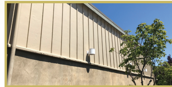
Repaired Dry Rot at Corte Madera School
