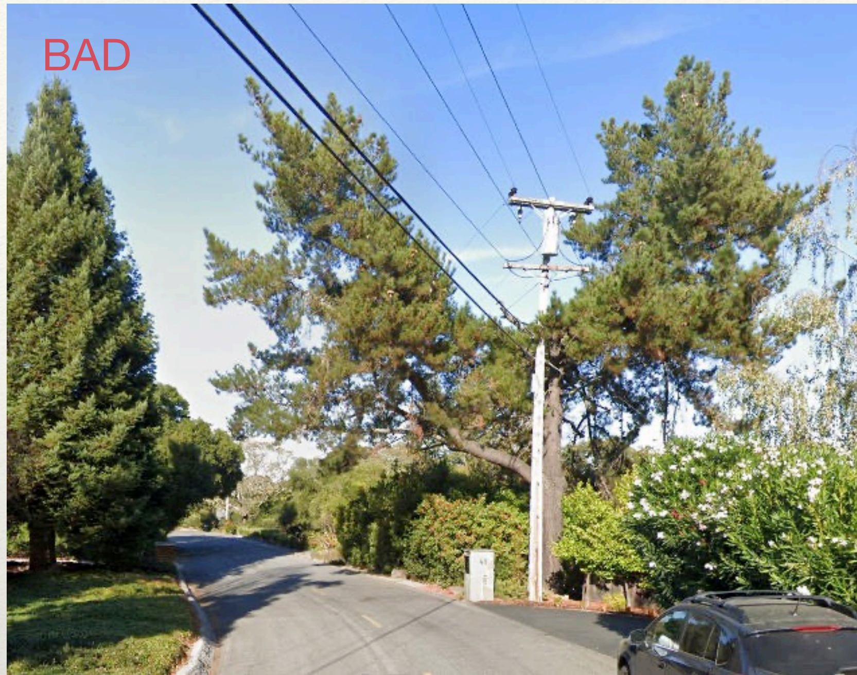
Overhanging Pine in Right of Way
