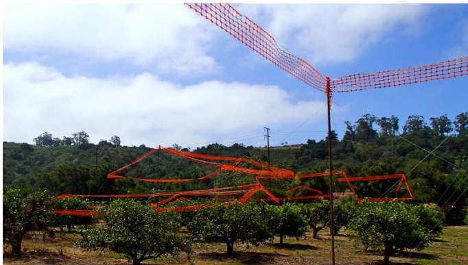
Figure 1. Story poles for a proposed single-family home located in Rancho Santa Fe, California.
