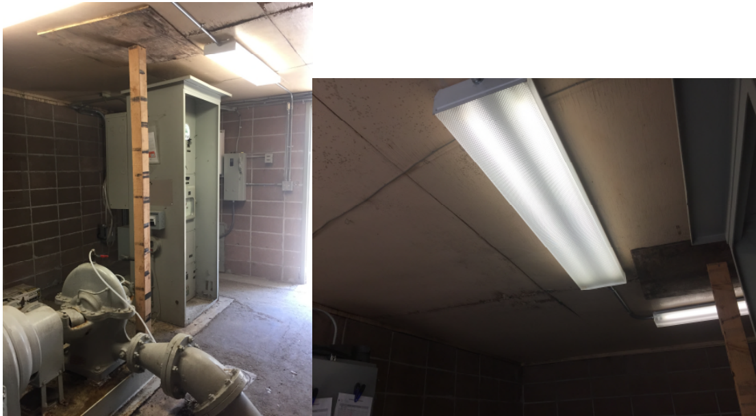
Photo 2 & 3) Photo of inside of building and support.
