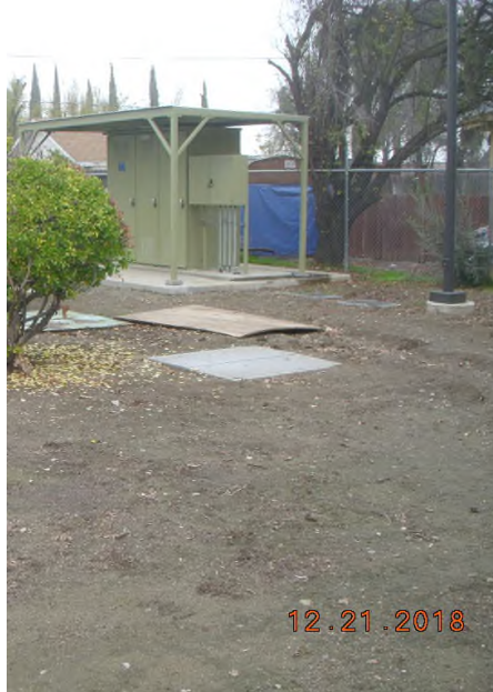
Photo 4 & 5) Photos of outdoor panelboard with shade structure. Awning can be attached to panelboard.
