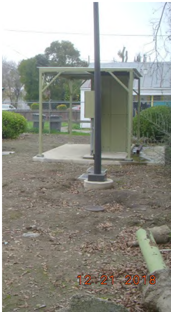
Photo 4 & 5) Photos of outdoor panelboard with shade structure. Awning can be attached to panelboard.
