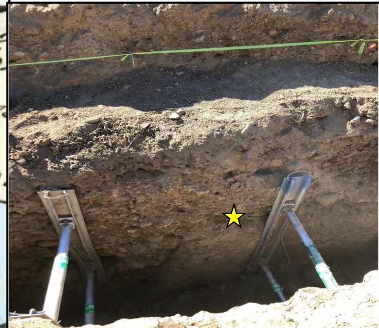
Trench Photo 35-40 ft
