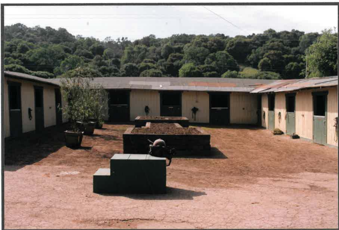
Photo 20. The roof was repaired, doors repaired or replaced. The inner yard walls were refaced and painted. A large perennial bed was established to organize traffic patterns.
