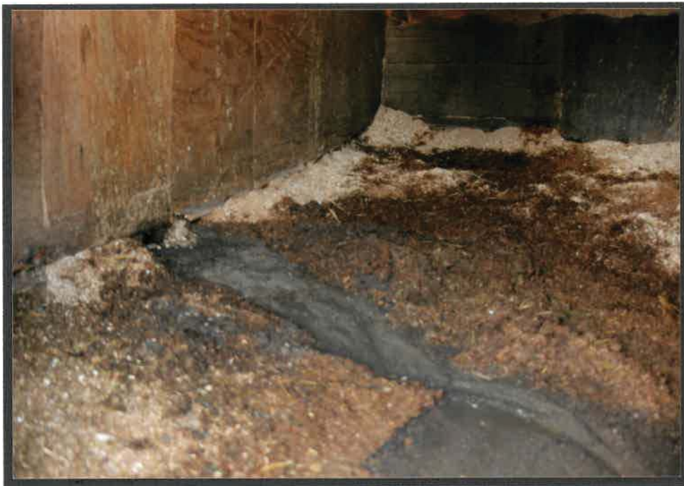
Photo 19. Drainage in the stalls was bad to non-existent. Some stalls had streams of water running through them.
