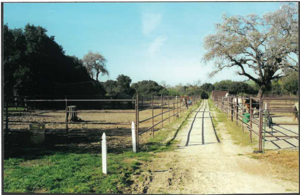
Photo 9. The new paddocks were built along a central lane to facilitate feeding and cleaning. Steel pipe panels were used to prevent chewing and the eliminate the need for nails that could hurt the animals, as well as for their strength and durability.
