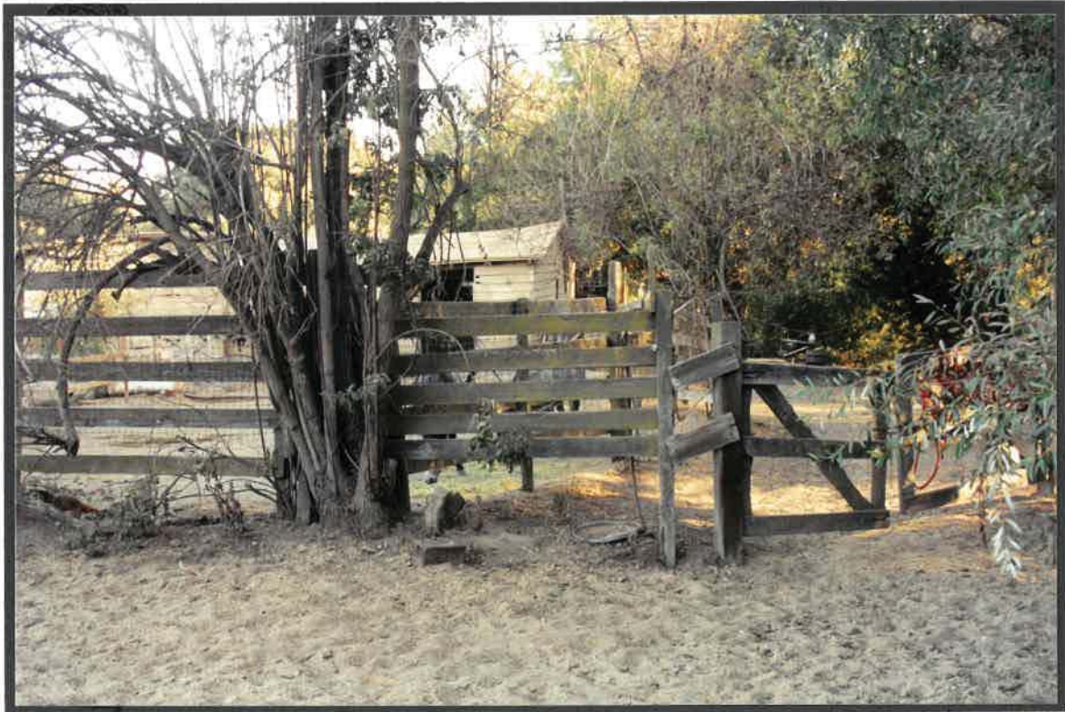
Photo 2. Wooden fences were in poor repair, gates insecure
