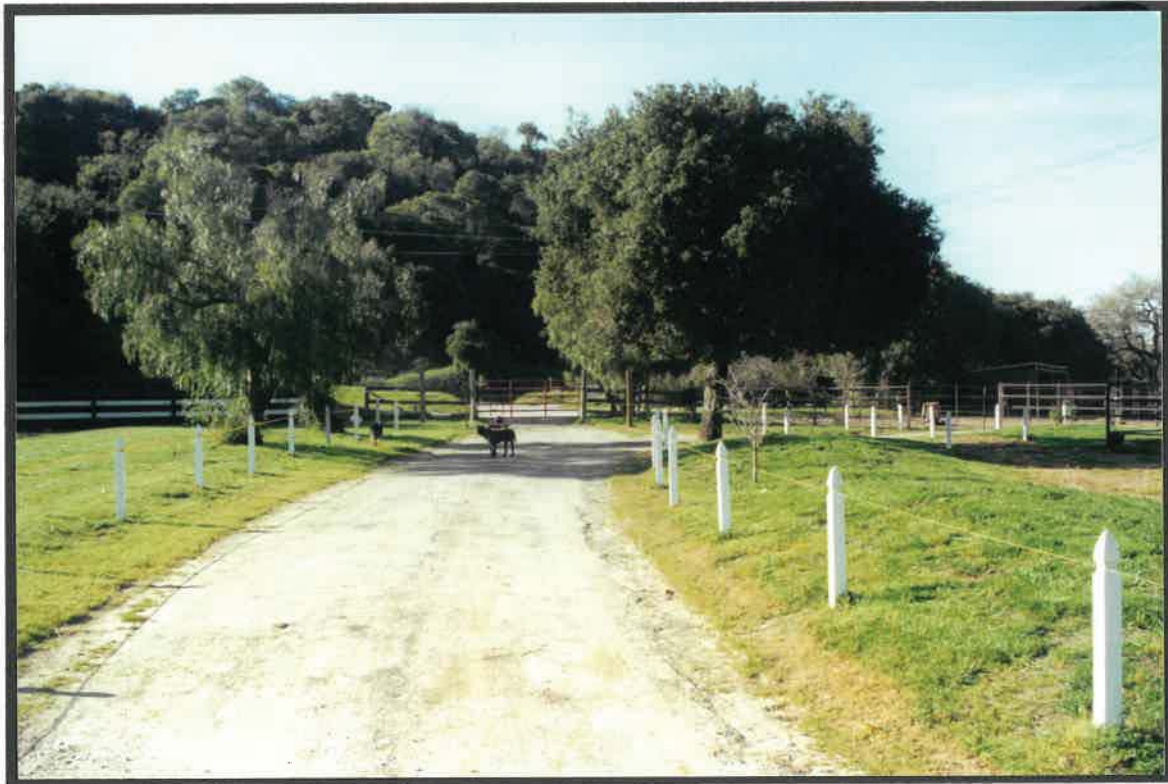
Photo 12. A broad open strip of land now borders the drive, opening up the view from the gate.
