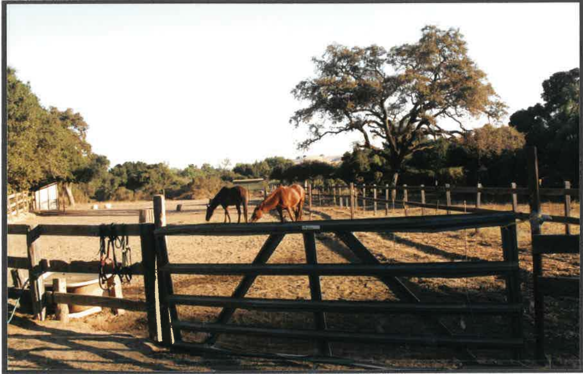
Photo 8. There were three large paddocks made largely of wire and steel posts. Where wood existed there were bare nails and broken boards. Leaking hoses and bath tubs were a constant source of water
