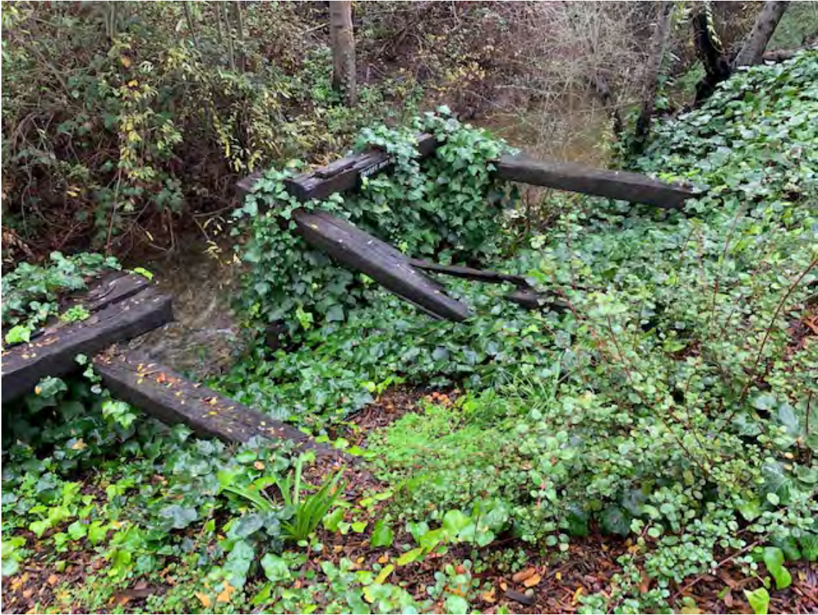
Photograph 1 – Railroad-tie ruins with vertical posts that are founded in the active creek channel.
