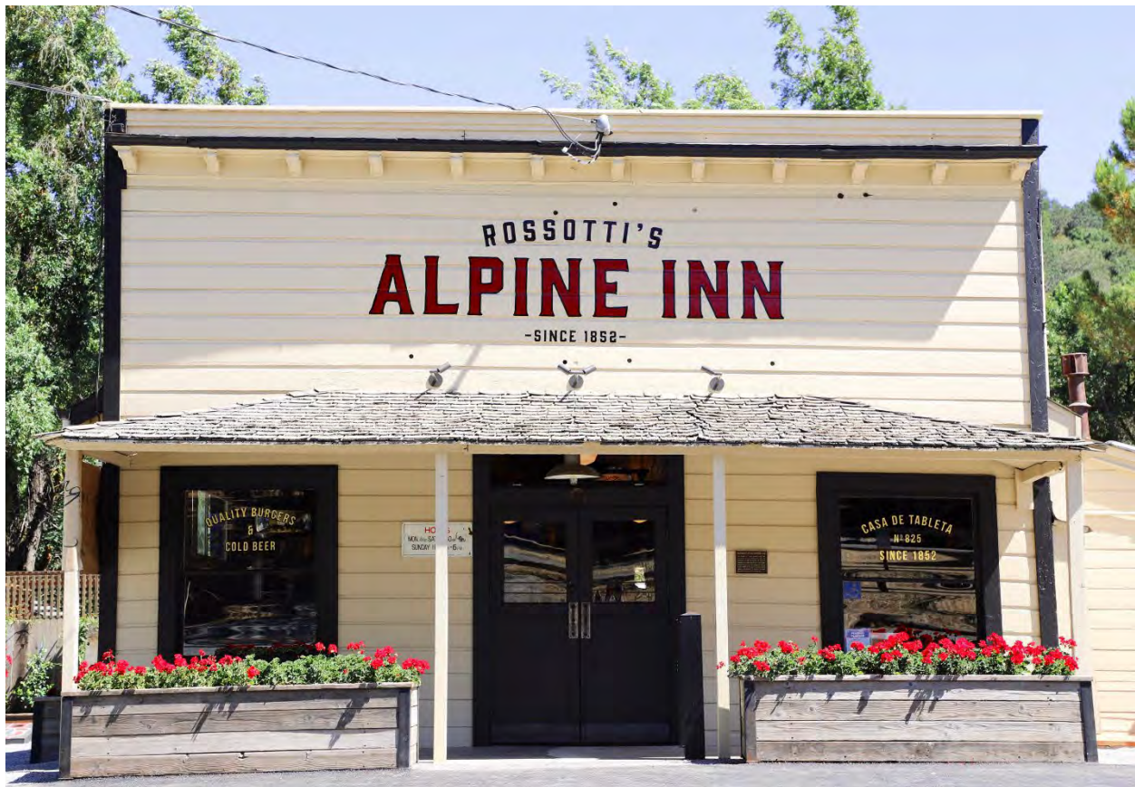
Figure 2: View of the primary façade of the historic portion of the Alpine Inn. Source: alpineinnpv.com
