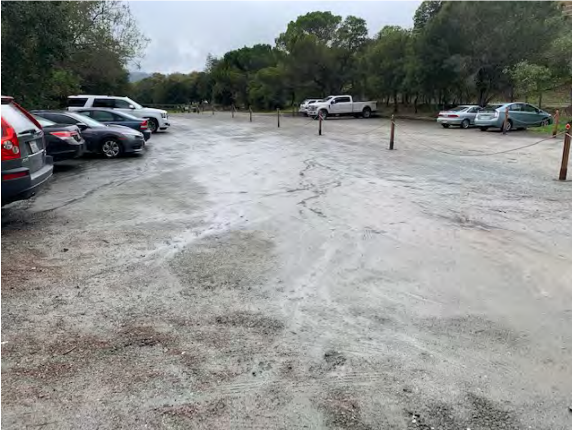
Photograph 3 – Runoff from the unpaved portion of the parking area feeds the erosion gully at the west end of the beer garden in Photograph 2.
