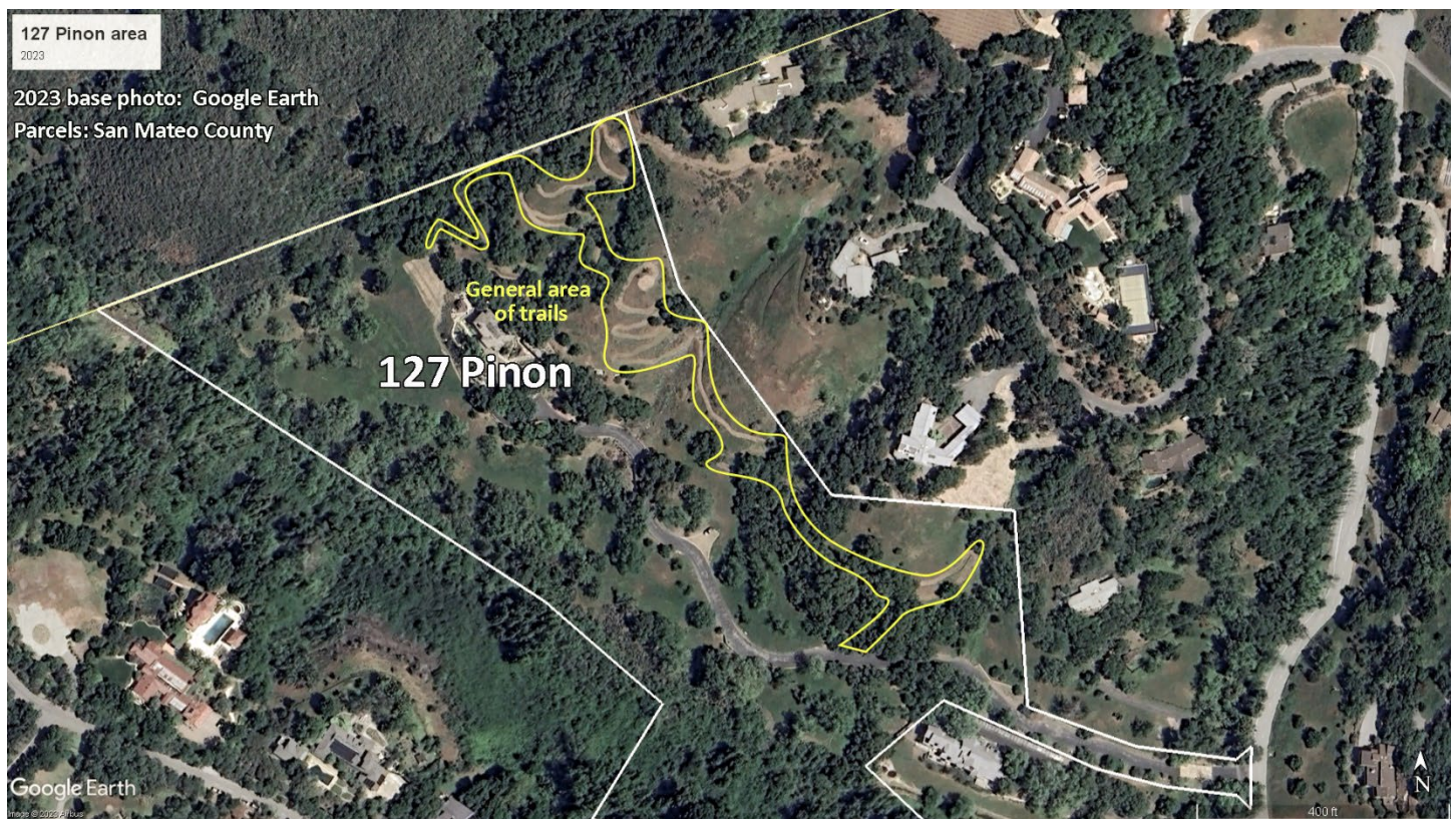
Figure 1. Aerial photo dated April 2023 (source = Google Earth) showing most of 127 Pinon, with parcel boundary (source = San Mateo County) in white. The yellow outline indicates roughly the areas of trail work and vegetation clearing or pruning based on aerial photographs from 2021 and 2023.
