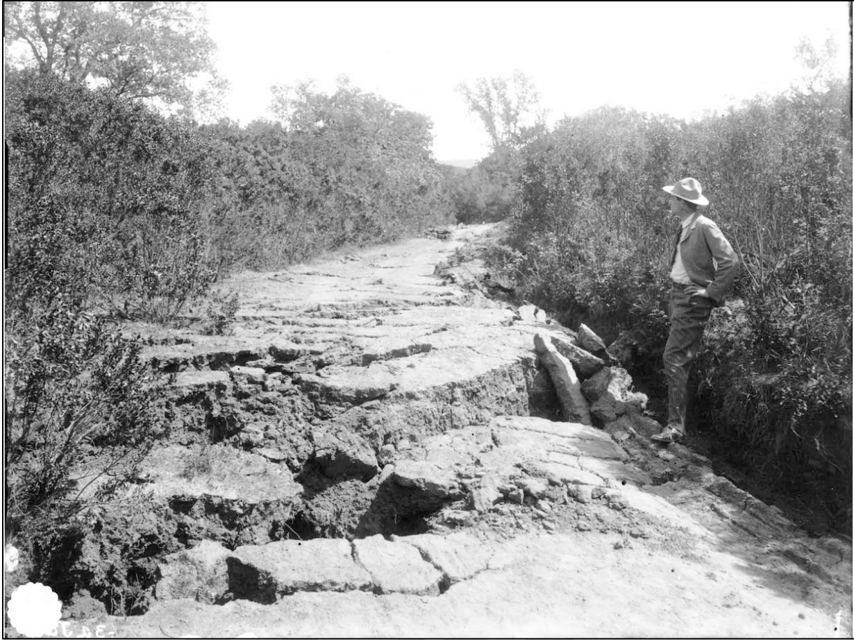
Figure 3. Vertical offset of Alpine Road 5 miles west of Stanford University. Per J. C. Branner. 1906 photograph from The California Earthquake of April 18, 1906: Report of the State Earthquake Investigation Commission (Lawson et al., 1908).
