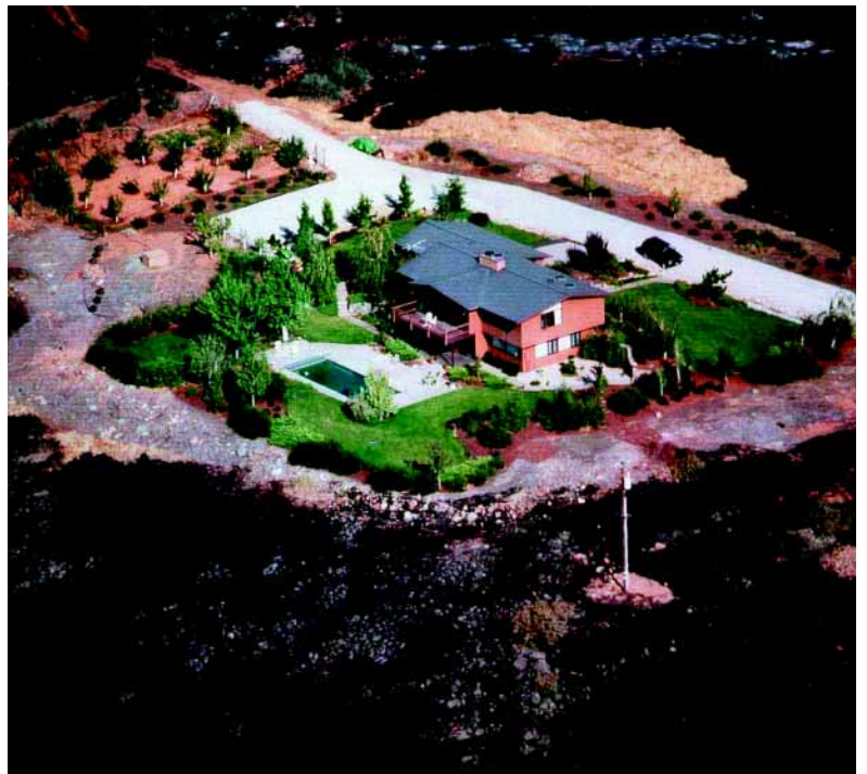
The pre-fire activities implemented by this homeowner included a green and well maintained landscape, reduction of wildland vegetation around the perimeter of the property, a fire resistant roof, and a good access road with a turnaround area. As seen in the photo, these pre-fire activities were effective.
