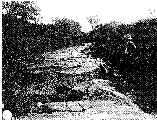
Figure 10. 1906 photograph to the southeast, showing the fault disruption at Alpine Road. The photograph, included in Lawson et al. (1908, plate 63A), was taken shortly after the earthquake. The fault broke along the south side of the road, as described by Branner (see text). Large fracture in the foreground is interpreted here as an en echelon fault break. This photograph was printed in reverse by Taylor et al. (1980).
