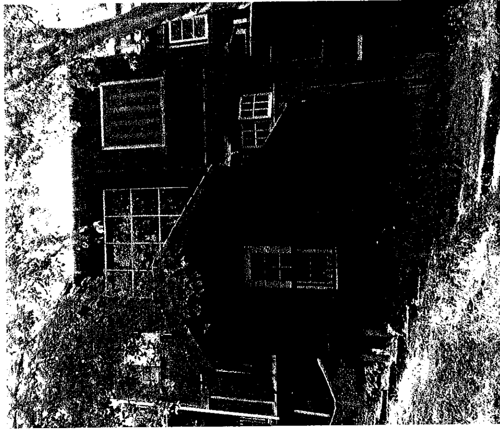
Image 6. South façade showing non-historic lower level porch with evidence of previous stairs and possible previous roof line, as well as non-historic square pane window and bay pushed out to roof eave.
