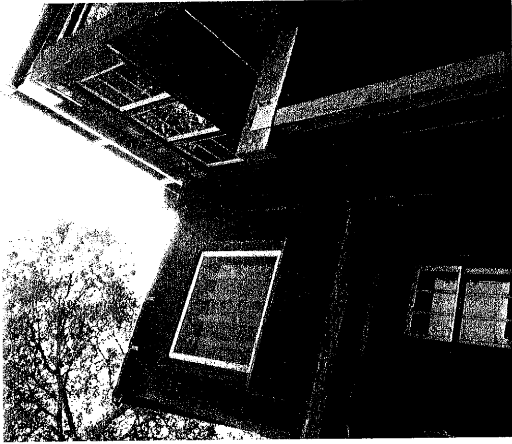
Image 7. East façade of area of proposed family room expansion, and south façade of non-historic addition.
