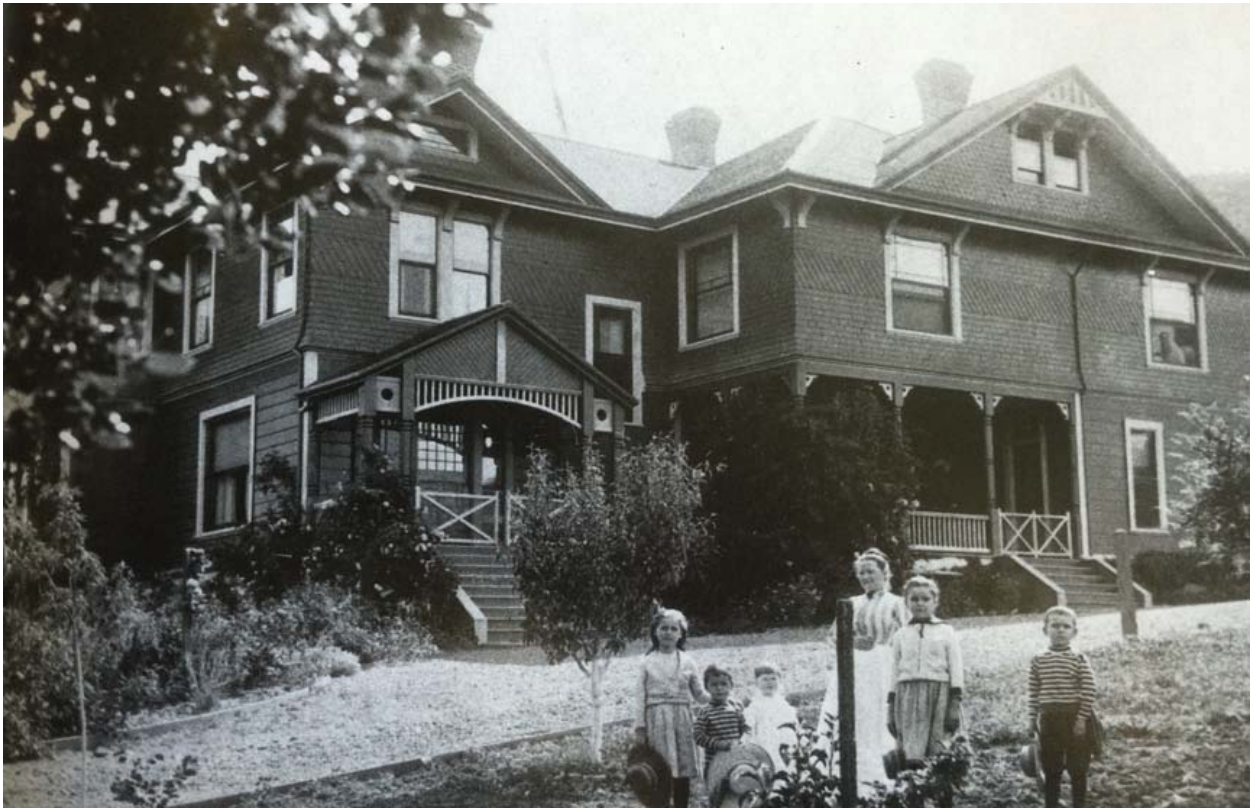
Hawthorn House, Allen era, north façade. Credit: G.T. White, 1893, Town of Portola Collection
