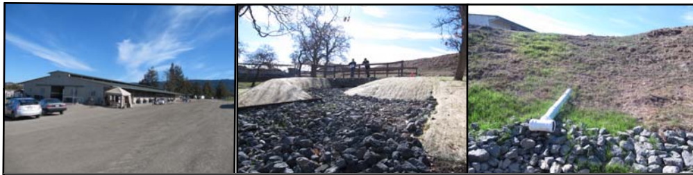
Left to right: building (20,000 sq. ft 2 ) with retention basin design; percolating section of the basin; and white, hillside drain directing storm water runoff into retention basin.
