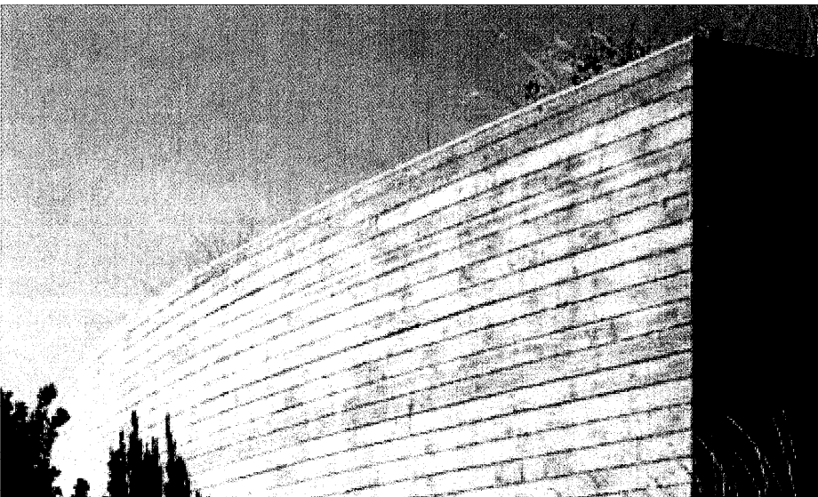
BOARD FORM CONCRETE WALL
