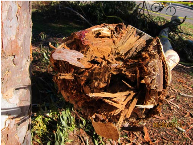
Branch end showing decay
