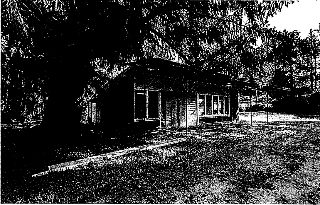
Sales office building, northwest and southwest facades (Architectural Resources Group, February 2016)
